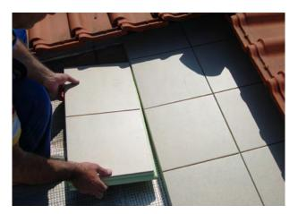
Fitting the insulating panels for better stability takes place by moving the first piece of every new line around 30cm. The correct jointing of the pieces is necessary.
