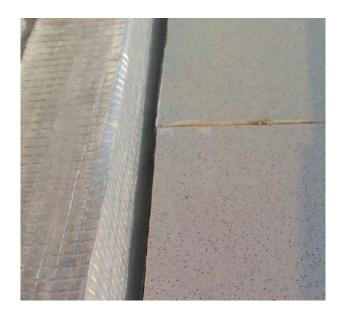
We make sure there is a joint of 2-3 cm from the original parapet (if there is no parapet, it must be built) and on the roof perimeter for the contraction and the expansion of the insulating panels. In case the roof is over  $50\text{m}^2$ , then an extra expansion joint should be maintained at the centre, with a width of 1-2 cm.
