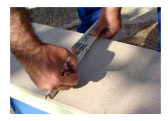
Careful study before the installation of **novablok Terrace** will ensure less cuts and waste. The application of tiles must take place on clean and even surfaces, always starting from the perimeter.
